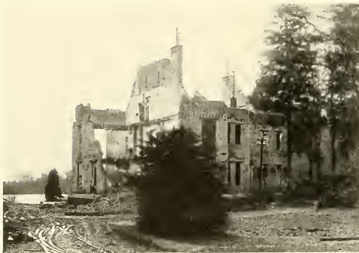
Only shattered walls left standing at LE NOUE LE COQ
